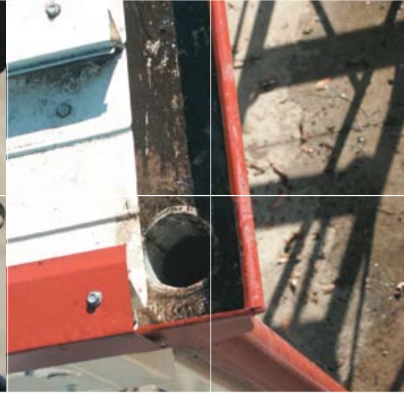
3) When litter is removed, the layer of hardened dirt is revealed below.
