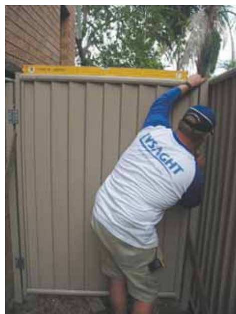
Figure 18.1 Fixing of hinges
