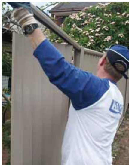
Lifting top rail helps ease 1st sheet into end position.
