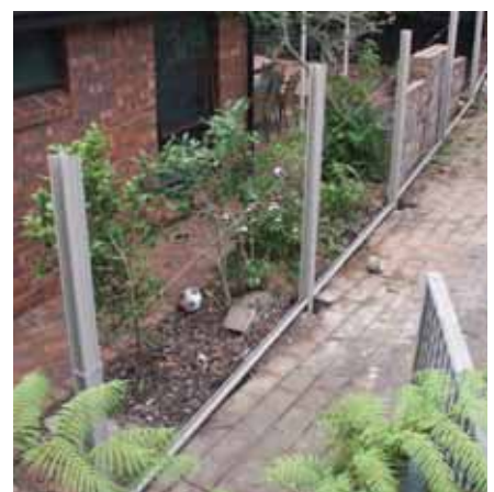
Set all the bottom rails into position ensuring a 50mm ground clearance.
