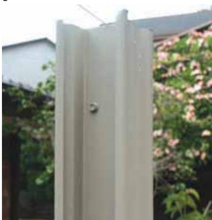
Use stringline to set post heights.
